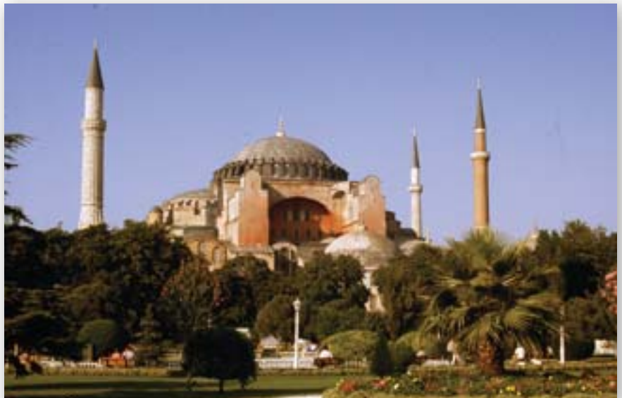
The members of the Fourth Crusade were astonished by the massive Hagia Sophia in Constantinople. The minarets date from after the Ottoman conquest. (Fred Nicolle photo)
